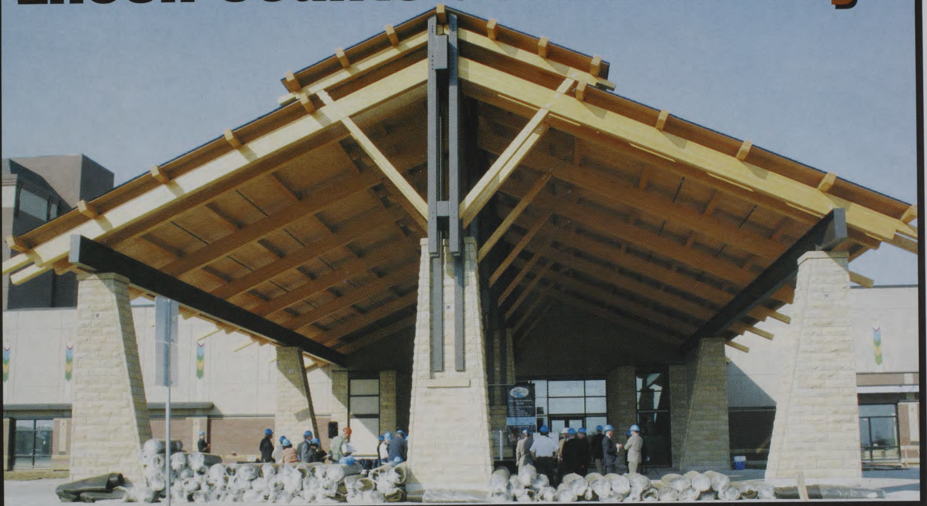
The canopy at the entranceway to the River Cree Resort and Casino was built large enough to accommodate the tour buses expected to journey to the site located on the fringes of Edmonton near West Edmonton Mall.
